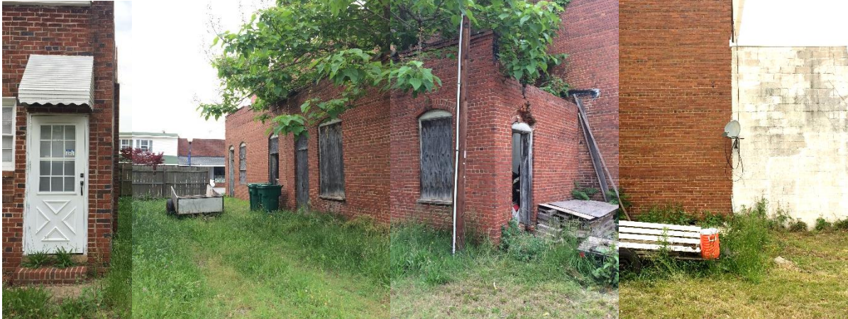
Back view of site showing two historic brick buildings to be preserved and repurposed.
